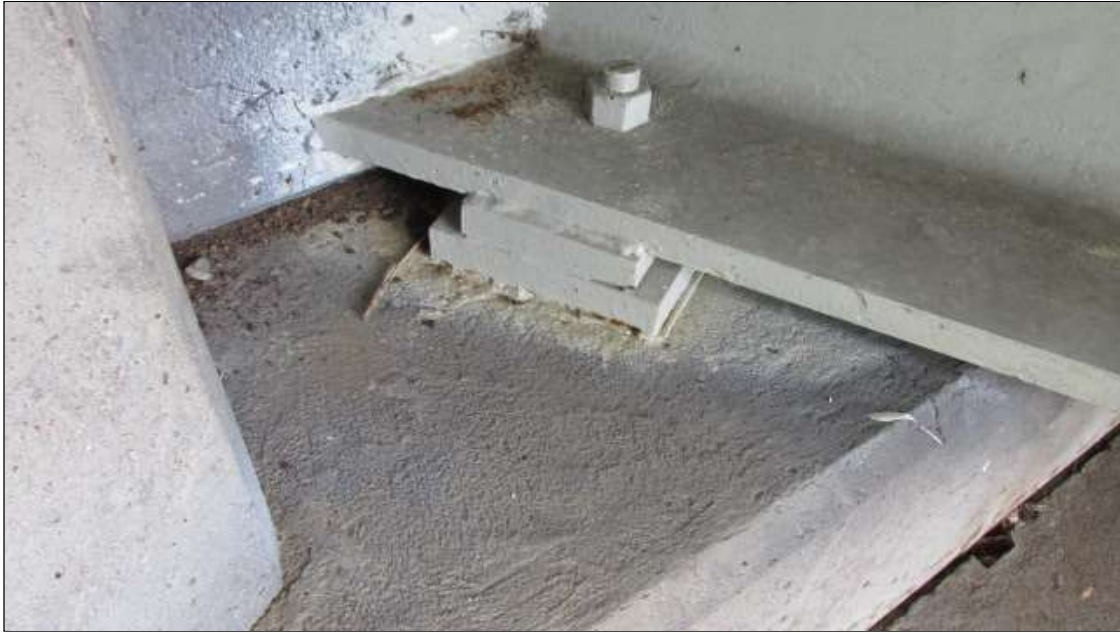
Span 1 Beam 6 Near Bearing : 1 Each of Corrosion: None. bearing painted
