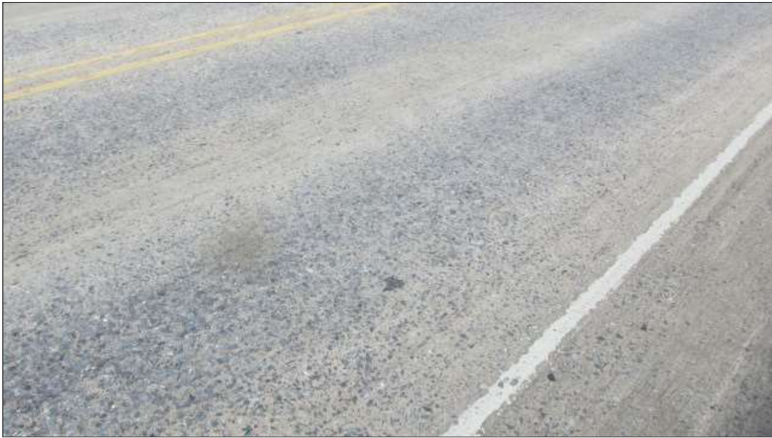
Span 3 Deck: 1500 Square Feet of Delamination/Spall/Patched Area: Delaminated. Spall 1 in. or less deep or 6 in. or less in diameter. Patched area that is sound.
