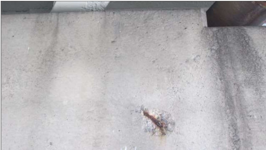
Bent 3 Cap : 1 Feet of Exposed Rebar: Present without measurable section loss. 6" diam. spall on the east face of cap under girder 2.
