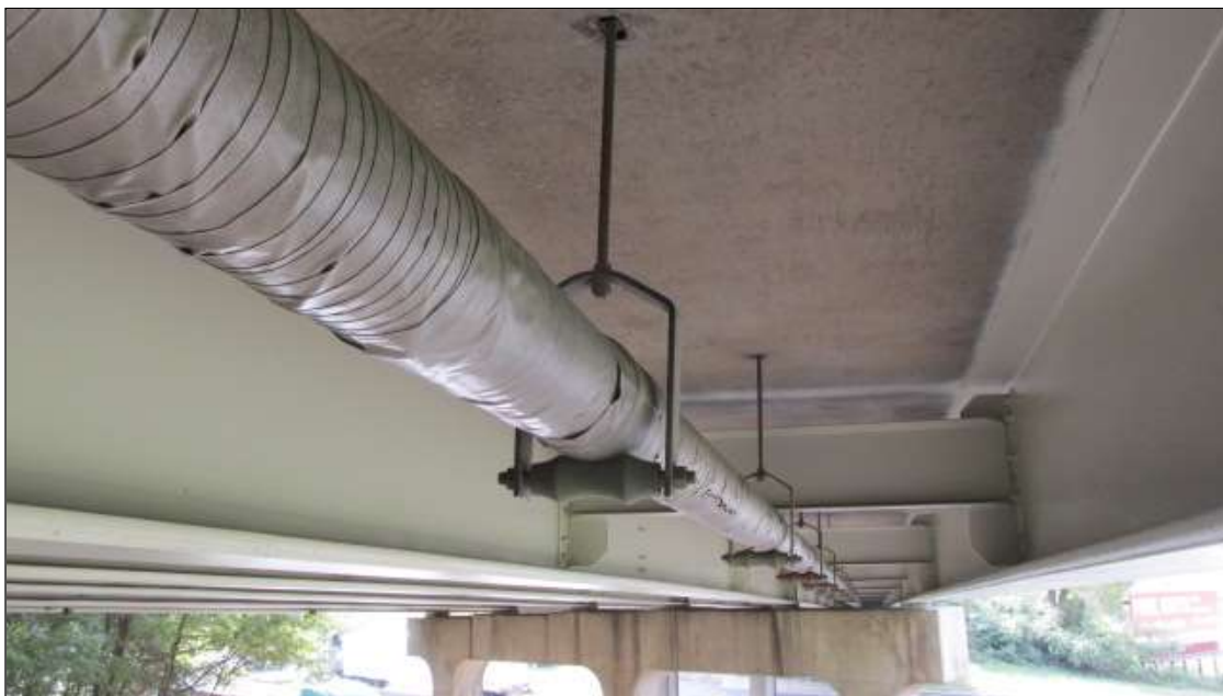
utility under bay 5
