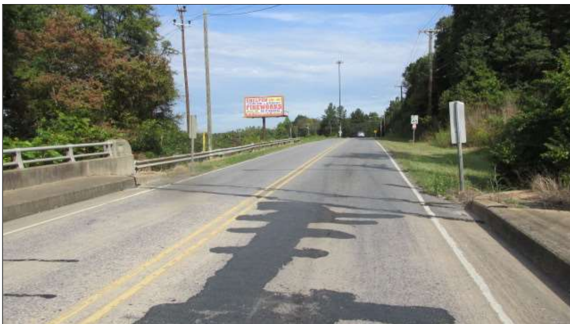
guardrail looking west
