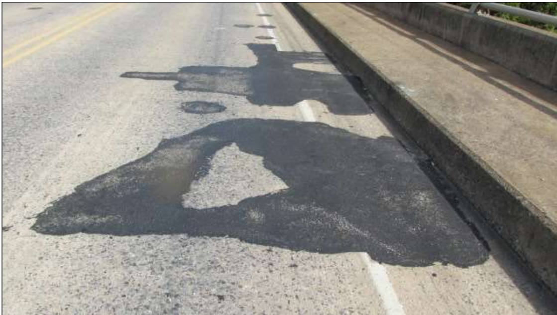
Span 2 Deck: 180 Square Feet of Delamination/Spall/Patched Area: Delaminated. Spall 1 in. or less deep or 6 in. or less in diameter. Patched area that is sound. a 20' x 6' wide asphalt patch in the lt. lane of span 2.
