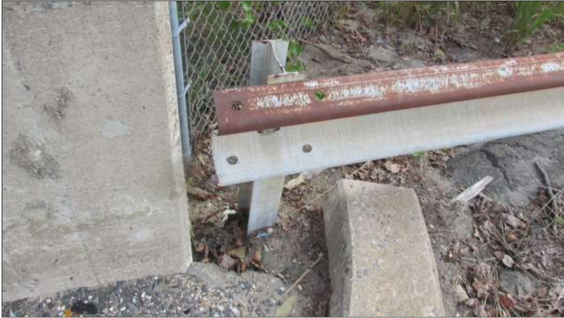
guardrail at the bridge for the ne and sw corners
