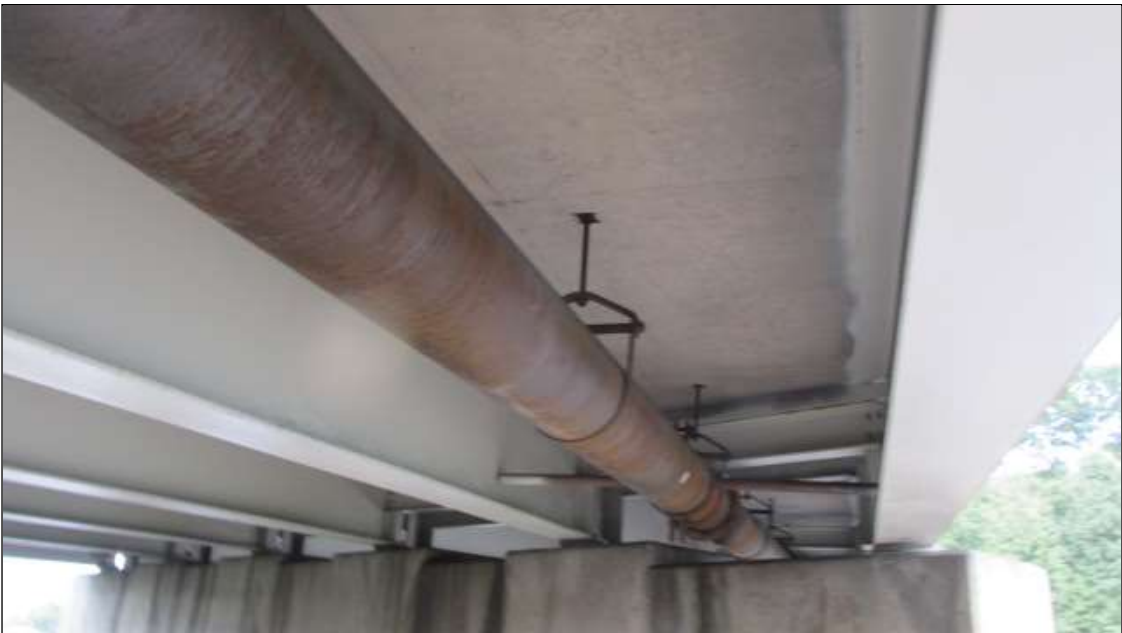
utility in bay 1
