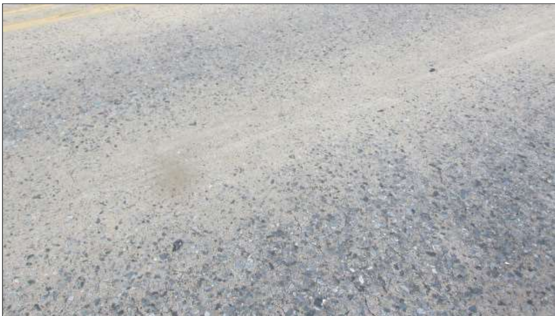
Span 1 Deck: 1000 Square Feet of Delamination/Spall/Patched Area: Delaminated. Spall 1 in. or less deep or 6 in. or less in diameter. Patched area that is sound.
