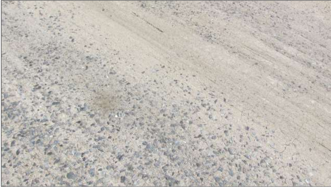
Span 2 Deck: 1000 Square Feet of Delamination/Spall/Patched Area: Delaminated. Spall 1 in. or less deep or 6 in. or less in diameter. Patched area that is sound.
