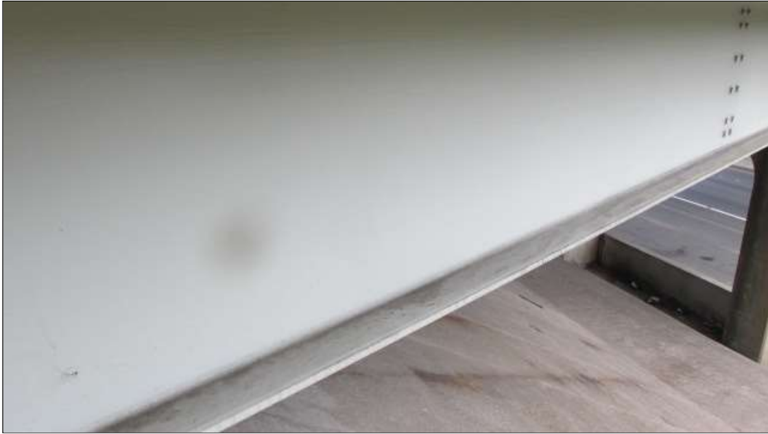
beams, bearing and diaphragms. painted recently
