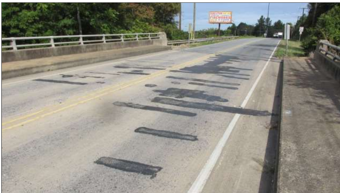
Span 1 Deck: 1000 Square Feet of Delamination/Spall/Patched Area: Delaminated. Spall 1 in. or less deep or 6 in. or less in diameter. Patched area that is sound. several patches in the lt. lane of span ranging from 1' x 2' to 6' x 10'.
