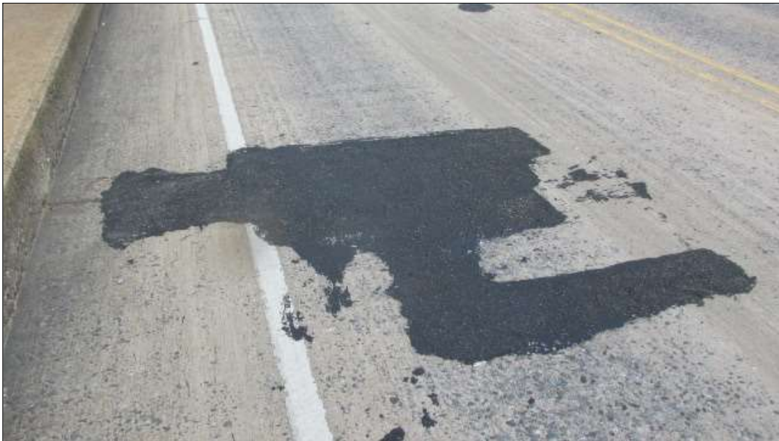
Span 2 Deck: 20 Square Feet of Delamination/Spall/Patched Area: Delaminated. Spall 1 in. or less deep or 6 in. or less in diameter. Patched area that is sound.. 5' l x 4' wide asphalt patch in the rt. lane
