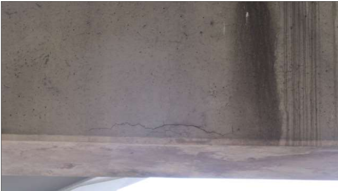
Bent 1 Cap : 3 Feet of Cracking (RC and Other): Width greater than 0.05 in. or spacing of less than 1 ft. west face bent
