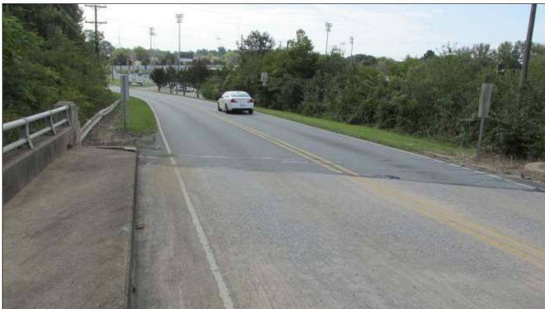
guardrail looking east
