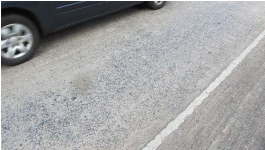
Span 4 Deck: 1000 Square Feet of Delamination/Spall/Patched Area: Delaminated. Spall 1 in. or less deep or 6 in. or less in diameter. Patched area that is sound.
