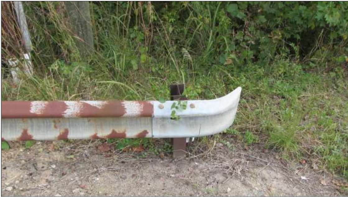
guardrail end at the sw and ne corners
